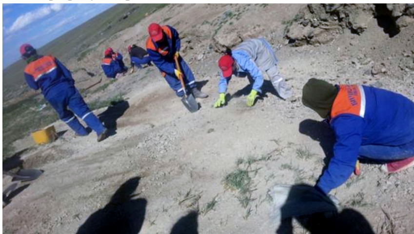
Picture 41: Holes were filled with waste material and compressed
