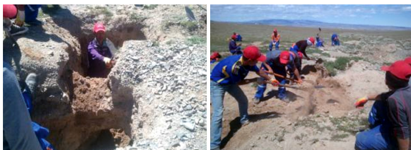
Picture 40: Holes were filled with boulders and rocks
