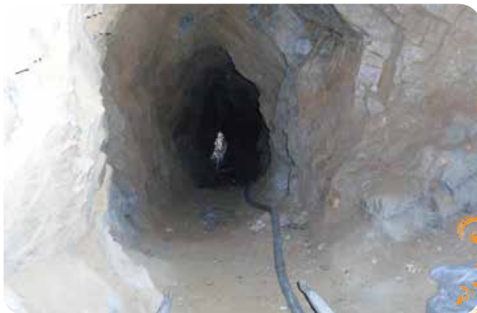
Photo 6: Constructing an adit shaft
