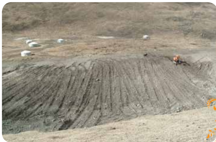
Photo 12: The process involved in undertaking technical rehabilitation
