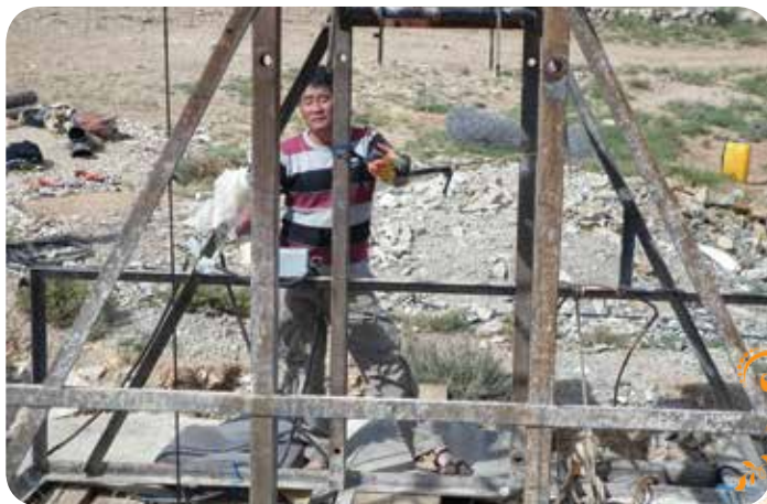
Photo 39: The communication system
