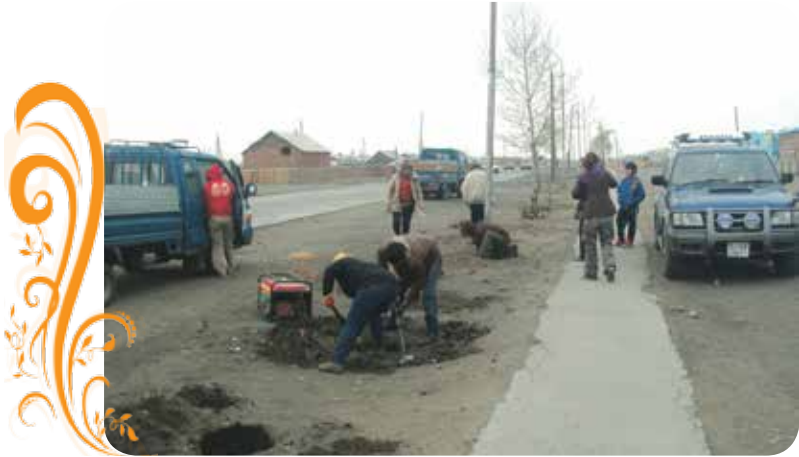
Photo 34: Digging holes for the planting of trees
