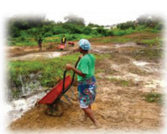
Figures 24 and 25: Former mine pits are filled in with nearby piles of overburden (left) and then converted into vegetable gardens and fish farms (right).
